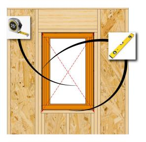
Place a level on the window sill to verify that the sill is level. Adjust the shims as needed to ensure a level condition. Check the head, sill and jambs with a level again to make sure the window is setting plumb, level, and square within the opening. Measure across the diagonals to determine if the window is square. Add shims around the entire window as needed to ensure a plumb, level, and square installation.
