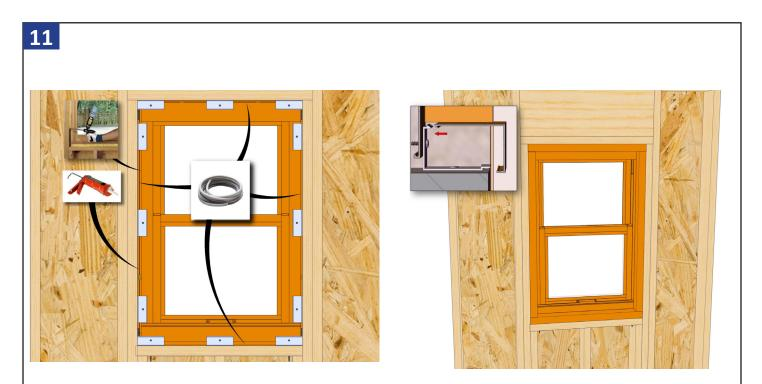
Insulate between the window frame and the rough opening using minimally expanding window and door spray foam or fiberglass insulation that is compliant with AAMA 812-04. Apply sealant continuously around entire perimeter of opening after foam or insulation is installed. Read and follow the manufacturers' recommendations for application and use. Measure and trim the snap covers to fit the opening, widths then heights. Install the snap trim covers to finish the interior.
