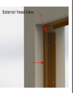
Shim as needed to level jamb receptor before tightening all screws. Apply sealant between receptor exterior and opening. Also seal both ends of head receptor to the opening.
