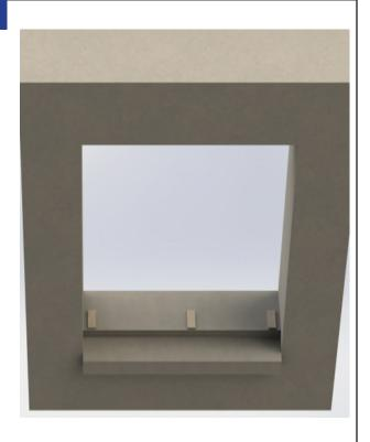
Check the fit of the unit making sure the conditions are level, the installer can pre-apply the shims to the sill condition prior to installation of the window frame.
