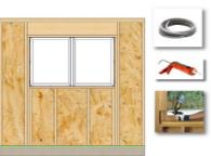
Insert the base plate with weather-strip flat against the window units and install with supplied bolts. Snap the finish trim cap over the base plate to finish the T-mull. Insulate and seal around the entire permiter of the window units.
