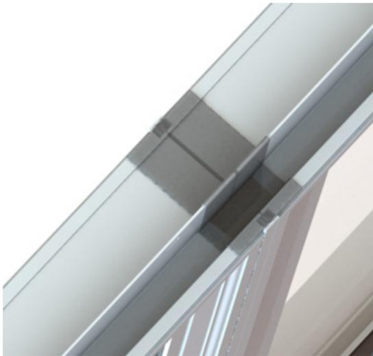
Seal both ends of the mull gaps with silicone the entire width of the frame covering any gaps.
